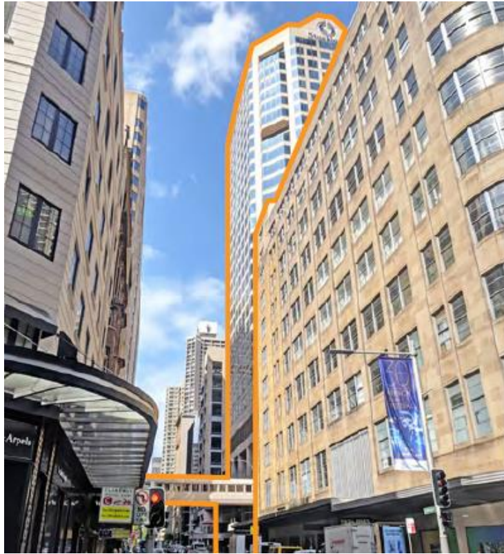
Figure 5. View along Castlereagh Street, looking south from Market Street
